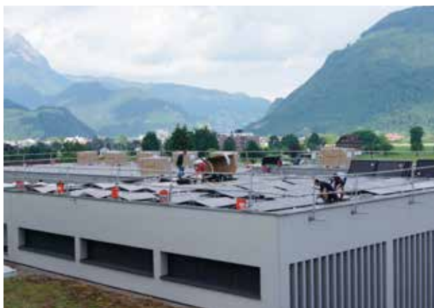
Installation der Photovoltaikpaneele
